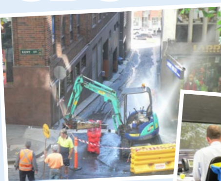
Michael Cambridge readies excavator for Level 2 demolition
